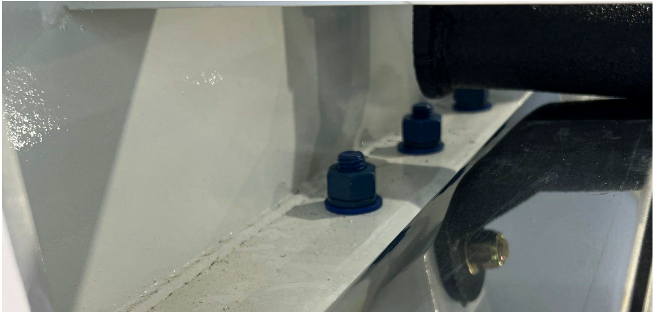
Figure 2: Upper Coupler Bolts
